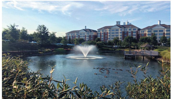
Photo Caption: Stormwater Management: Proactive stormwater management techniques can help improve the health of a community watershed and the beauty of the surrounding ecosystem.
